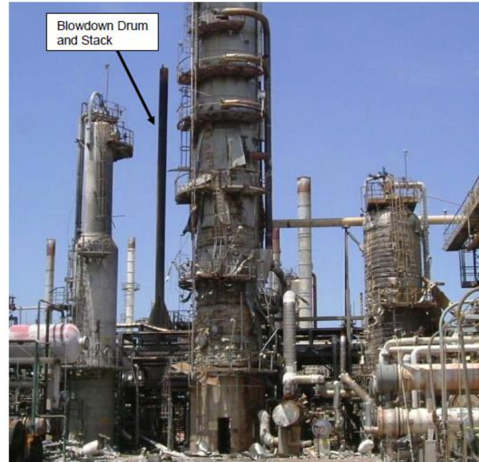
Raffinate splitter, after the accident
