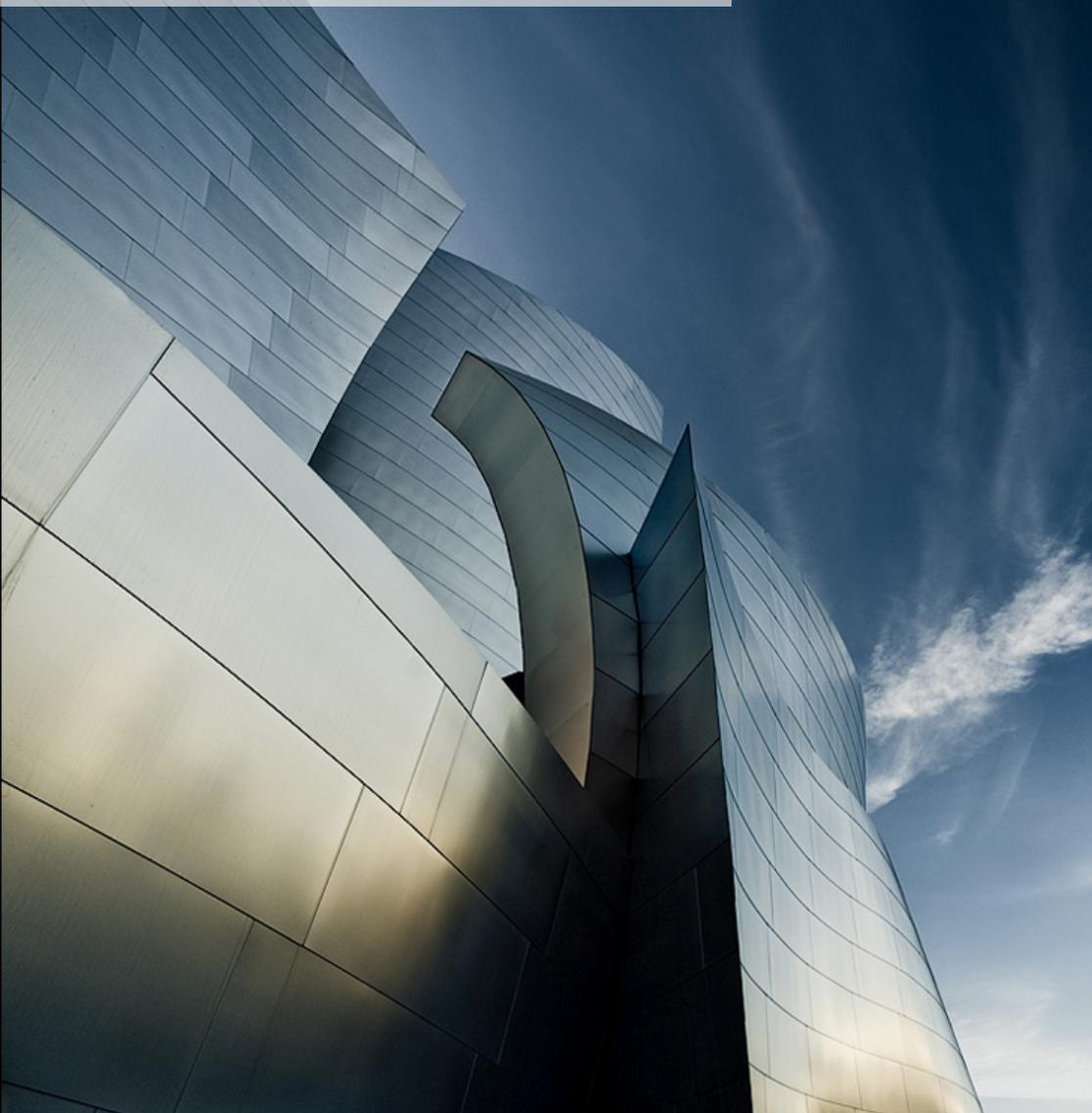
The cartographic problem of distortion is immanent to the construction of curvilinear architecture. Most building material is planar. This means only surfaces that can be mapped without any distortion – so called developable surfaces - can be fabricated and assembled relatively easy.
