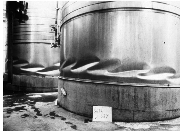
Buckled wine tanks. https://shellbuckling.com
