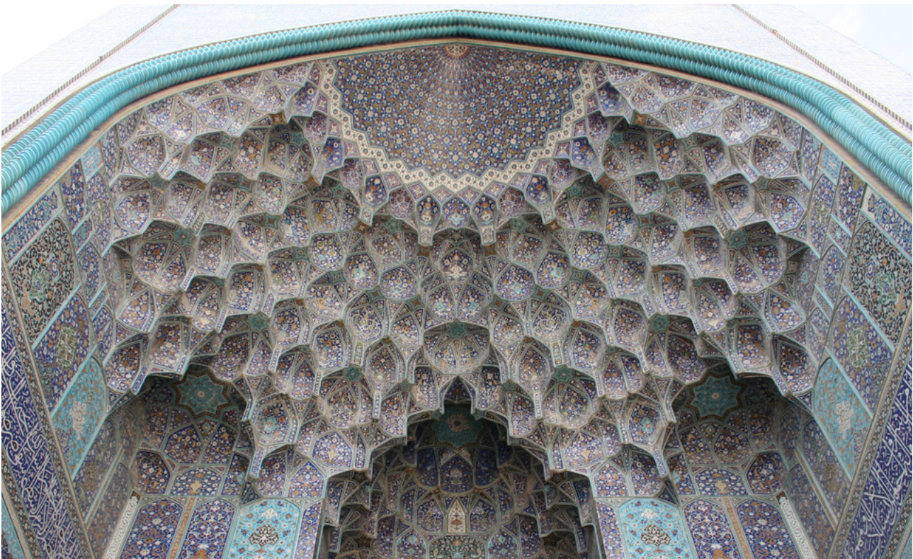
Fig.3.24. "Muqarnas", Complex geometries of Isfahan's Royal Mosque's Muqarnas and tile work comprises of patterns which are repeated in the space.
