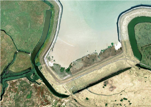
Fig.9.1. Site aerial view
