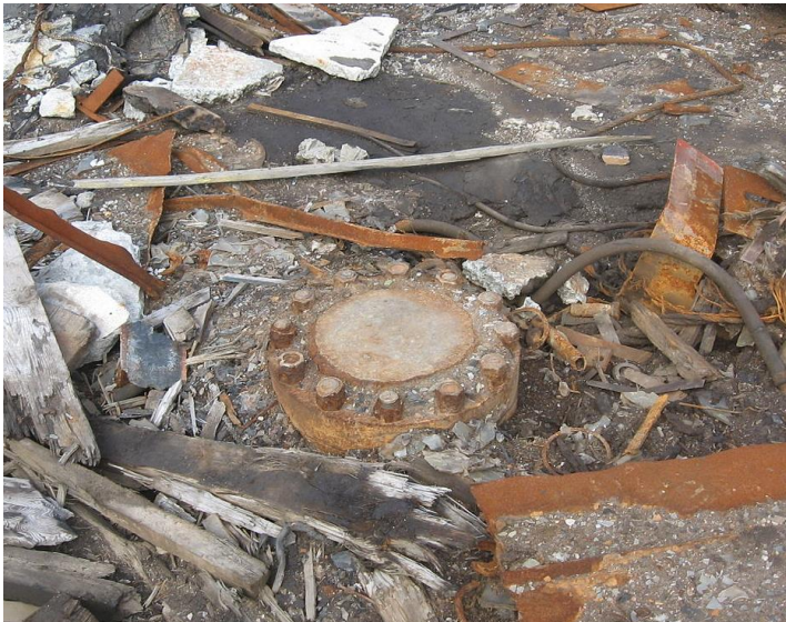
The borehole, welded shut
