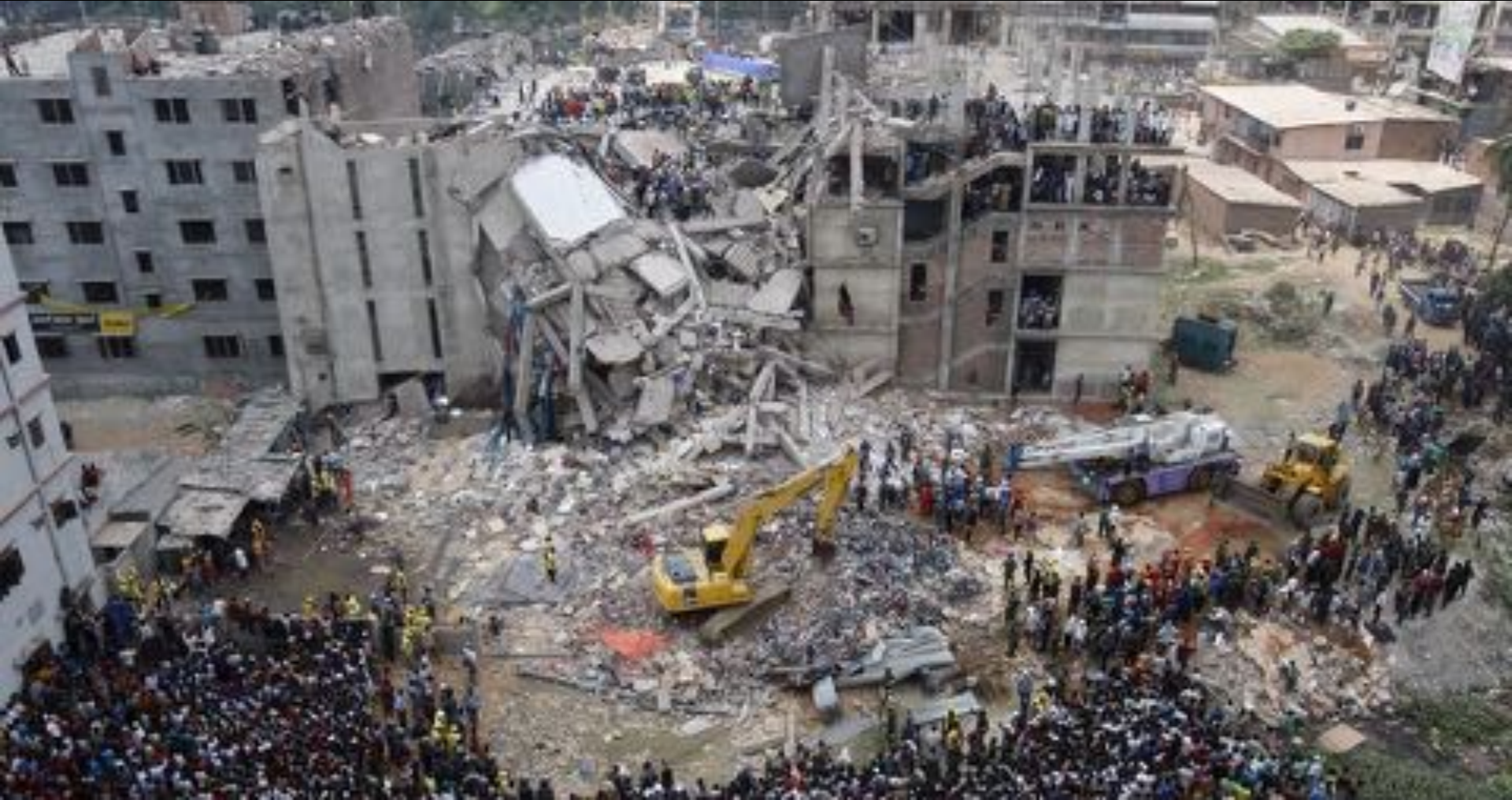
The collapse of Rana Plaza clothing factory 24.4. 2013. Over 3000 people killed or injured. Photograph: Abir Abdullah / EPA.
