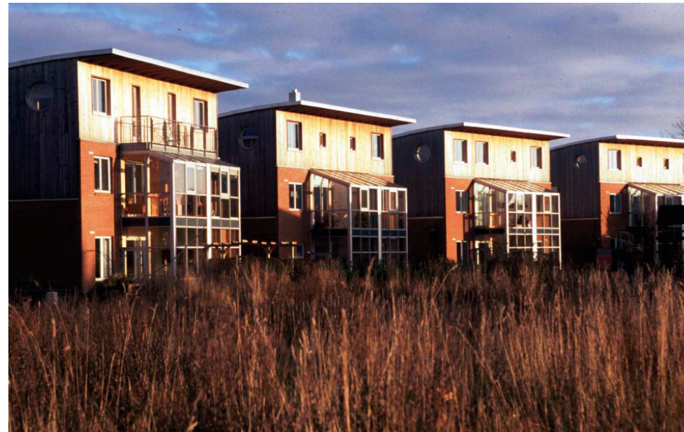
Fig. 4.18 Flintenbreite, Lübeck, Germany. Wetlands purifying greywater from a housing block. Blackwater is used to produce biogas.
