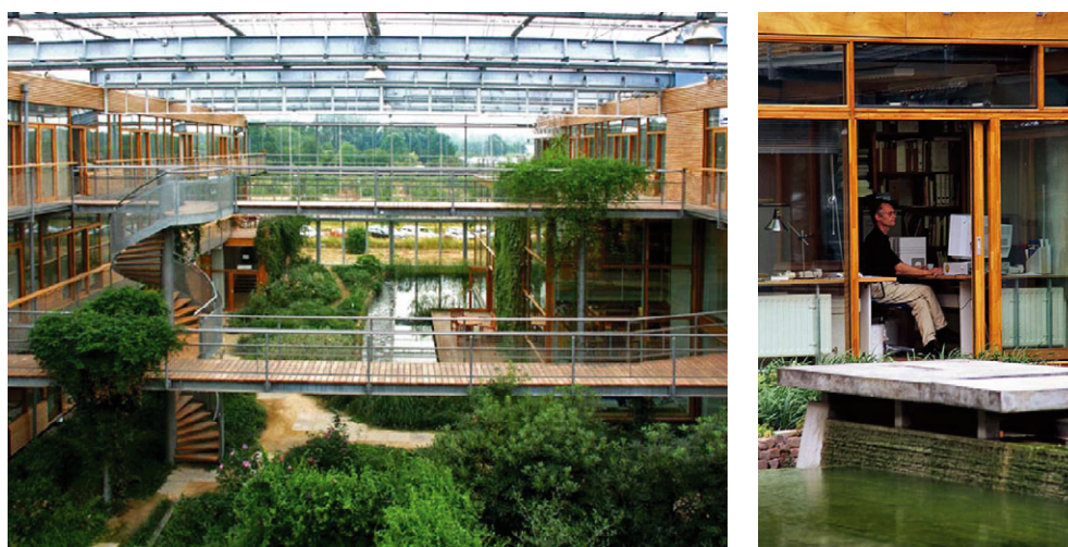
Fig. 5.38 Reference, courtyard: Institute for Forestry & Nature Research, Wageningen, the Netherlands. Architect: Behnisch & partners.
