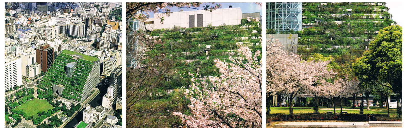
Fig. 5.34 Reference, terraces. Acros Building, Fukuoka, Japan. Architect: Emilio Ambasz.
