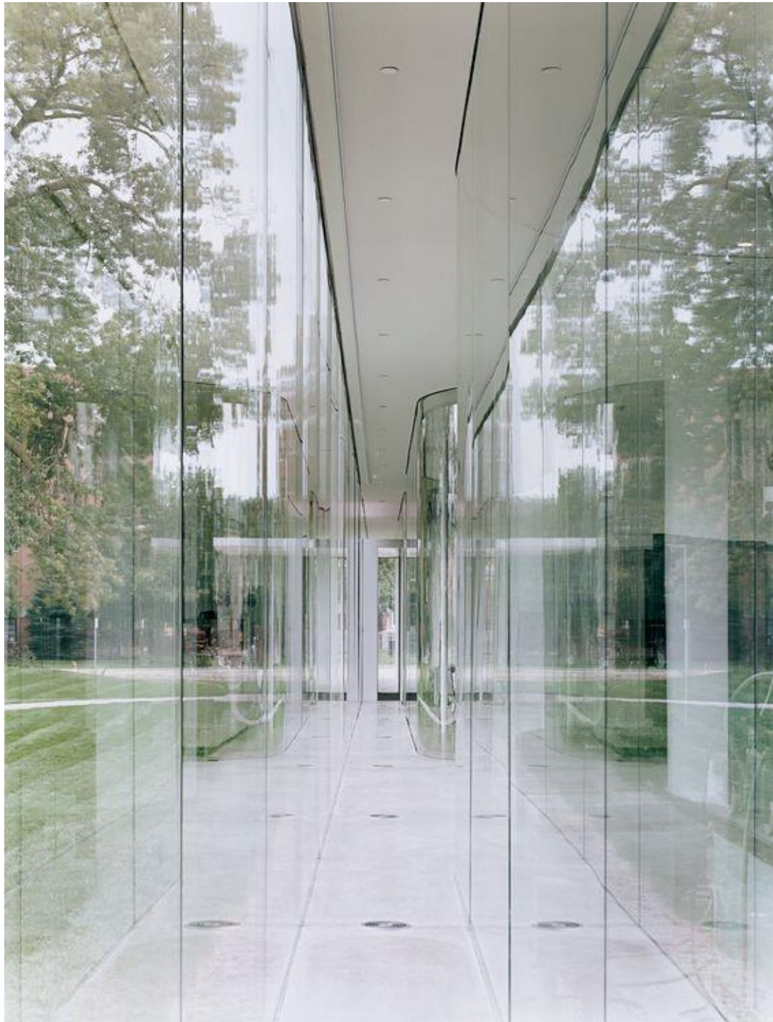
SANAA . Sejima and Nishizawa and Associates / The Glass pavilion . Toledo museum of art 2006
