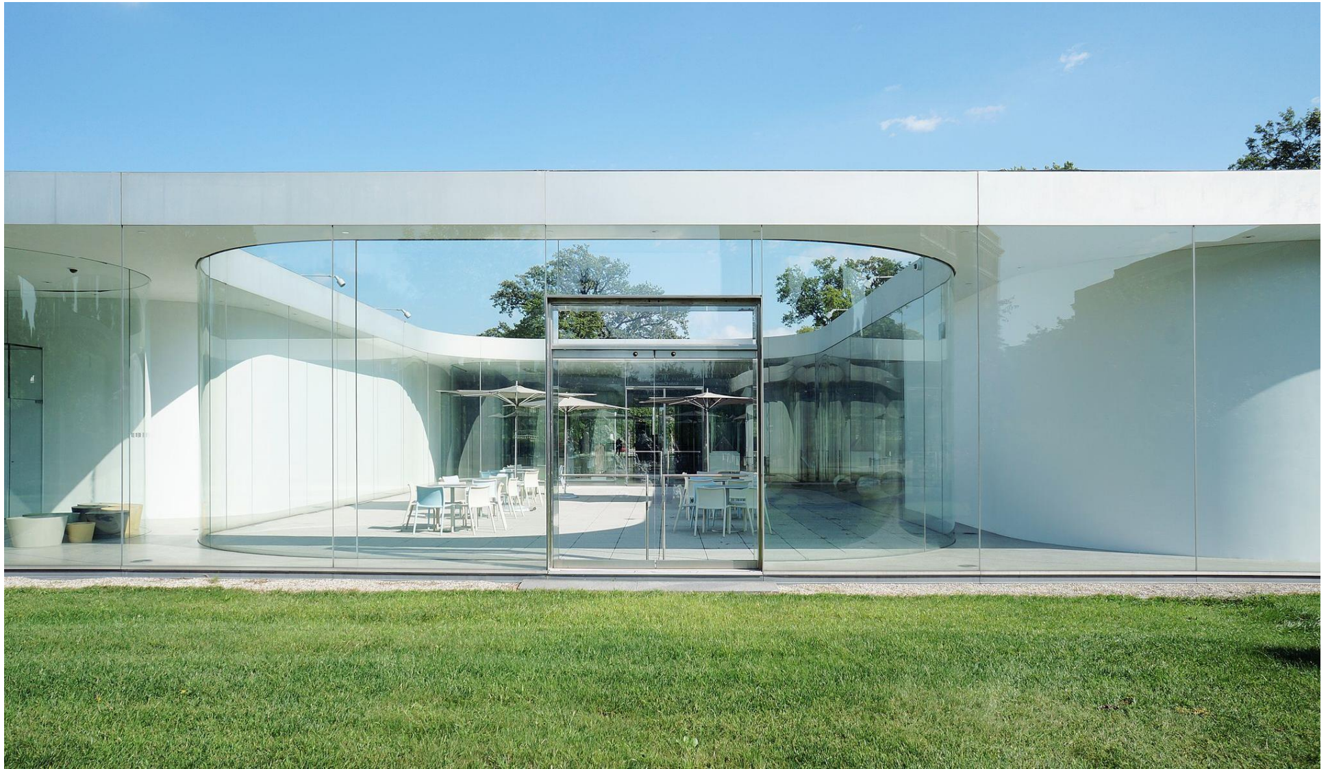
SANAA . Sejima and Nishizawa and Associates / The Glass pavilion . Toledo museum of art 2006
