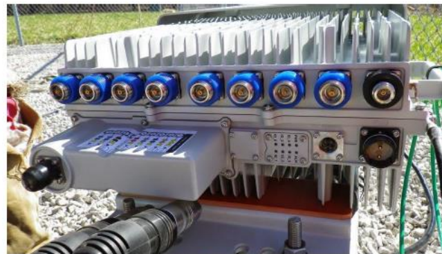
Sprint/SAMSUNG 8T8R installation
