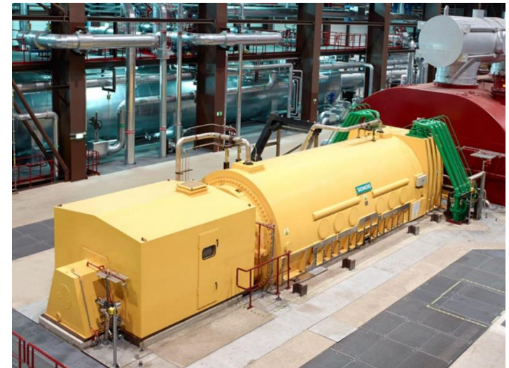
Generator, P = \sim 800 MW
