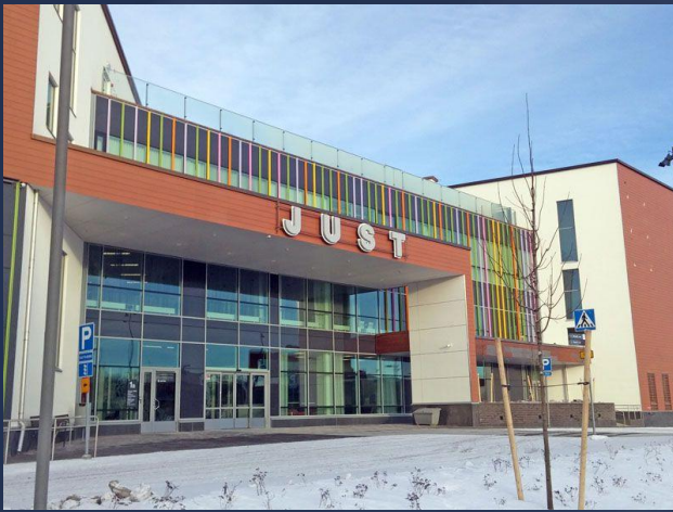
Järvenpää social and health centre (completed in 2017)
