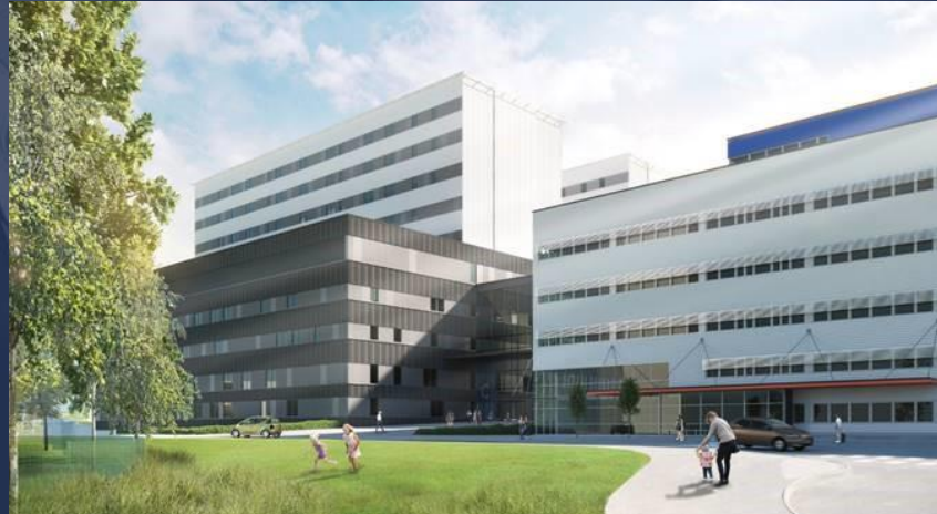
Oulu University hospital – OYS 2030 future hospital
