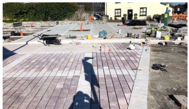
Civilised street under construction with raised bus kerb
