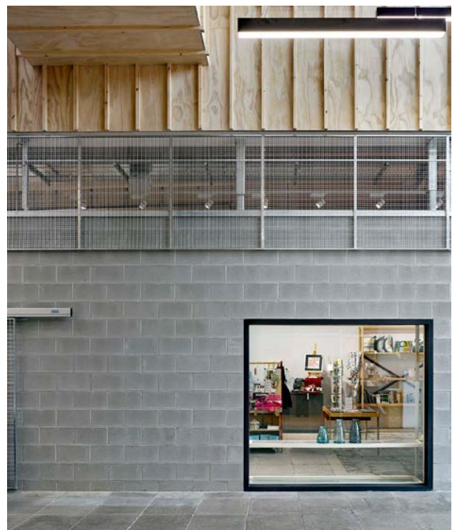
Exposing the structure
