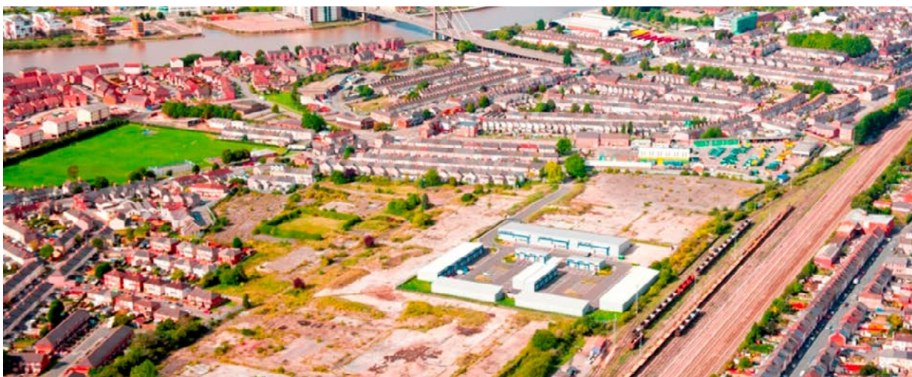
Aerial photo of the site before construction
