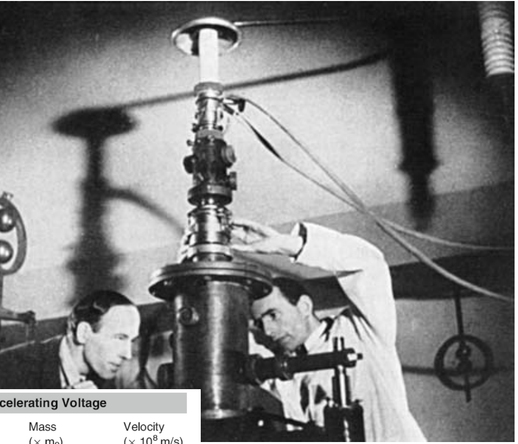
FIGURE 1.1. The electron microscope built by Ruska (in the lab coat) and Knoll, in Berlin in the early 1930s.
