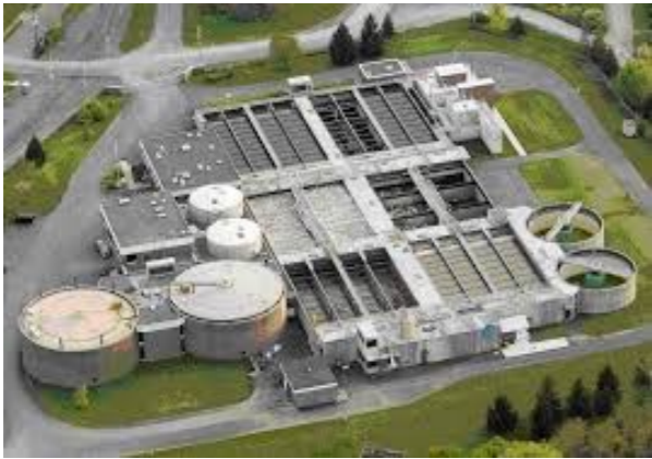
Waste treatment facility
