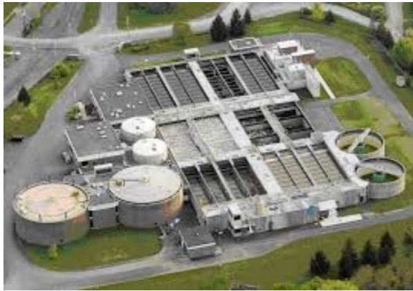
Waste treatment facility
