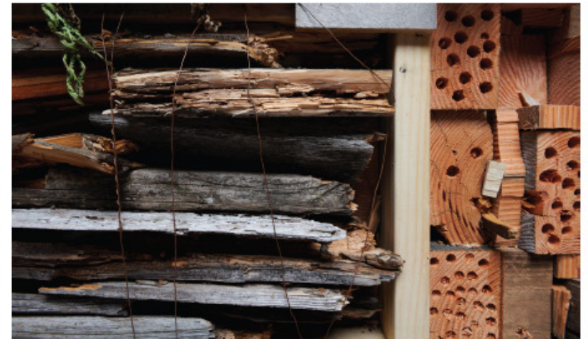
Figure 3/ Panel, or insect hotel, made from various materials includ- ing accoya and reclaimed wood.
