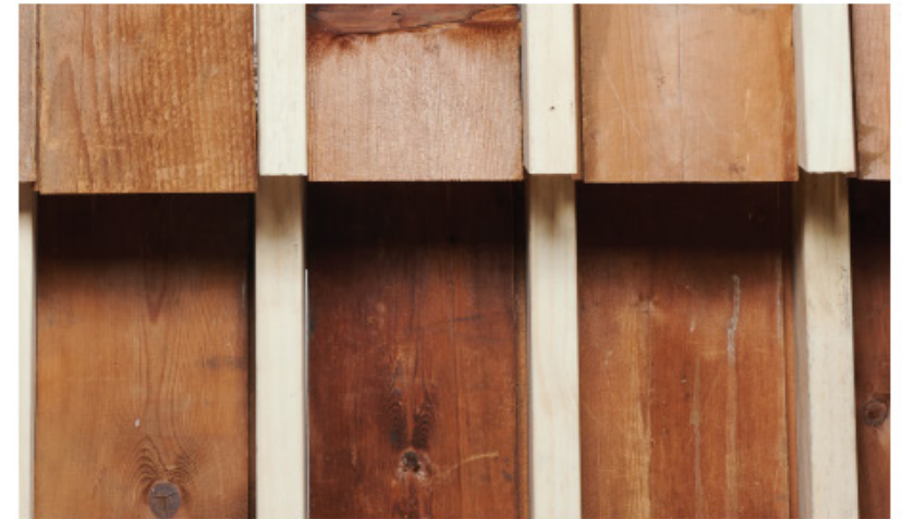
Figure 3/ Panel made from reclaimed floorboards and accoya..
