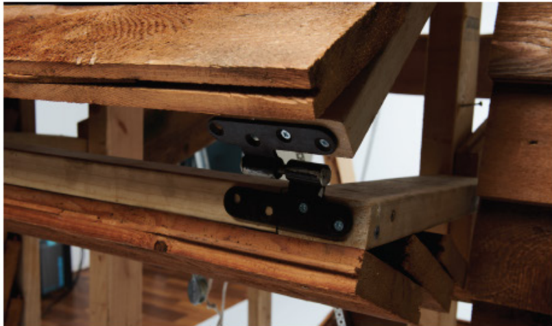
Figure 1/ Panel made from reclaimed floor- boards.
