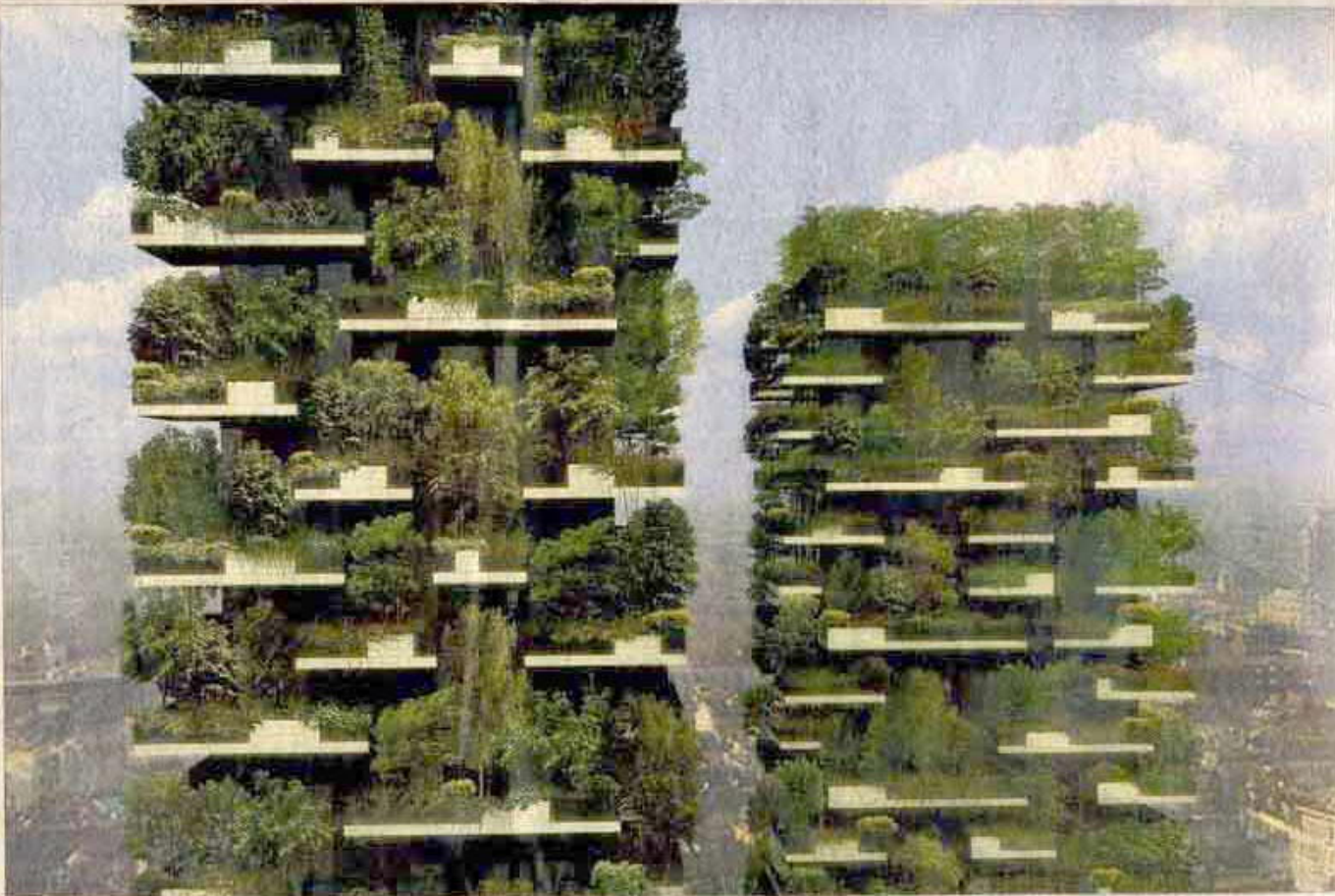
Above: the 27-storey Bosco Verticale in Milan, designed by Stefano Boeri as the world's first 'vertical forest'
