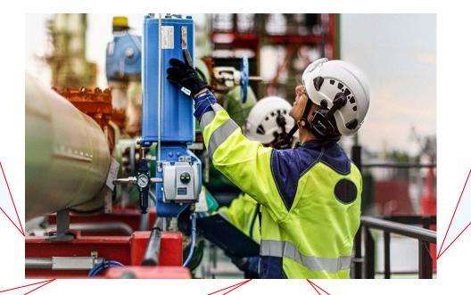
Preparation of the field box for check-out by clean blow of pneumatics etc.
