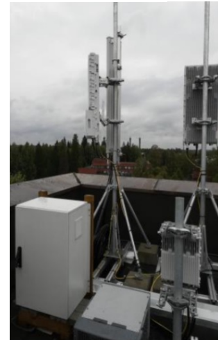
Aalto's 5G gNB on the roof of Väre building
