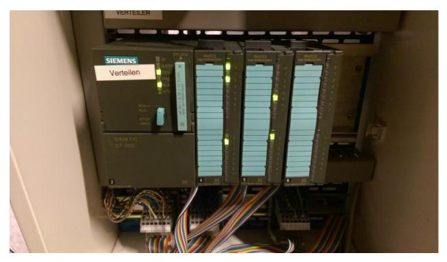
Figure 3 Siemens S7-314 PLC with three DIDO modules
