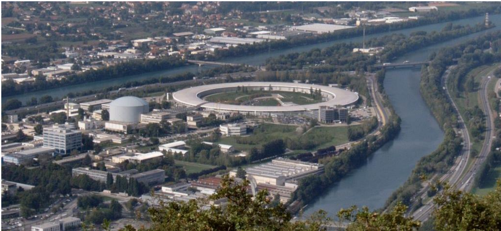
European Synchrotron Radiation Facility (ESRF) in Grenoble
