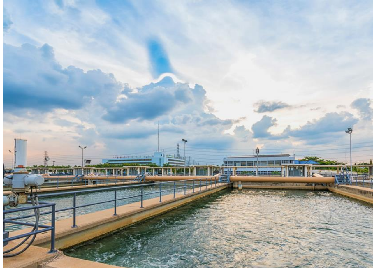
Municipal waste water treatment plant in UK
