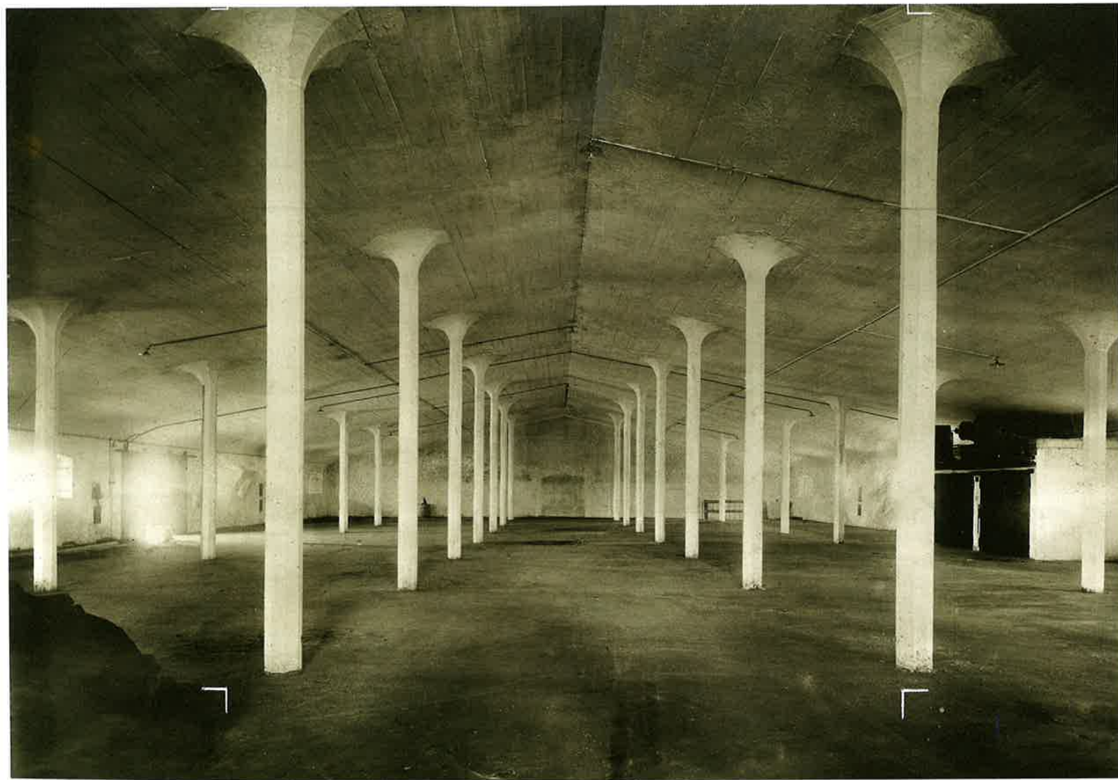
Warehouse in St. Petersburg by Maillart & Co., 1912
