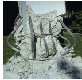
Kimmoton nurjahdus Inelastic buckling
