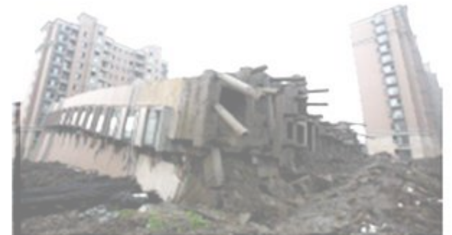
Soil material instability
