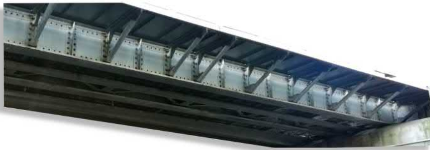
Figure 1.157: Old heavy railway bridge (Lyon, FR). Example of web stiffeners.
