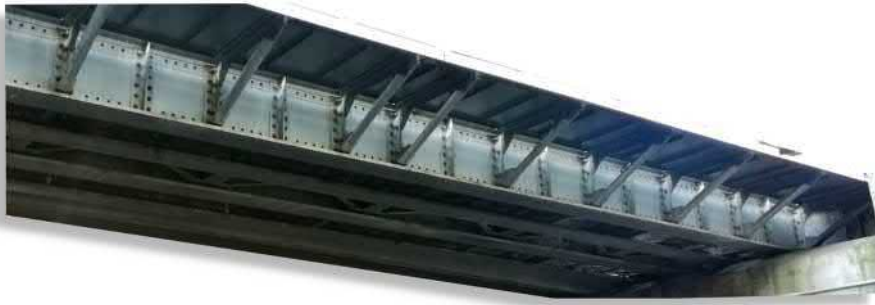
Figure 1.159: Old heavy railway bridge (Lyon, FR). Example of web stiffeners.
