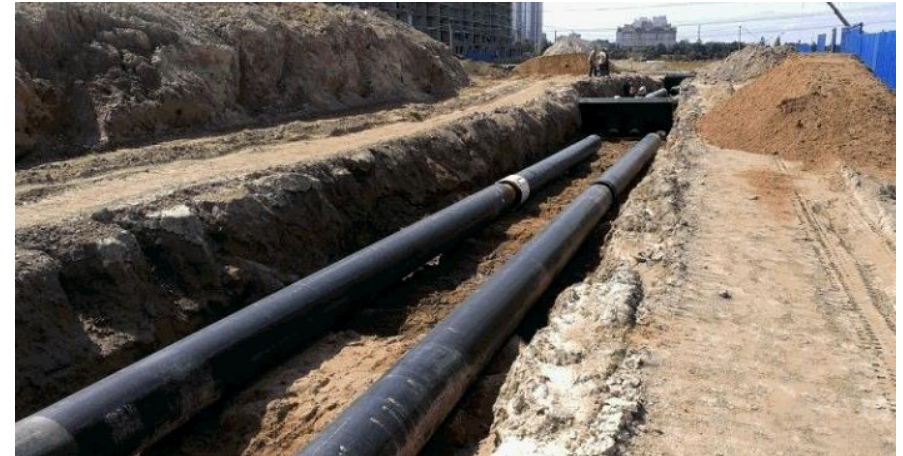
Buried Pipe Element (Underground piping) from https://www.passuite.com/kbase/doc/start/WebHelp_en/pipesoil.htm
