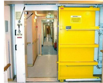
Watertight door. Image credit marineandoffshoreinsight.com
