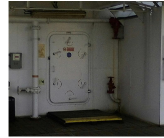
Weathertight door. Image credit marineandoffshoreinsight.com
