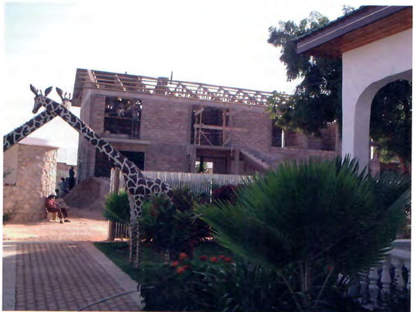
Figure 1.6 Roof trusses are more commonly used in Tanzania than in Madagascar
