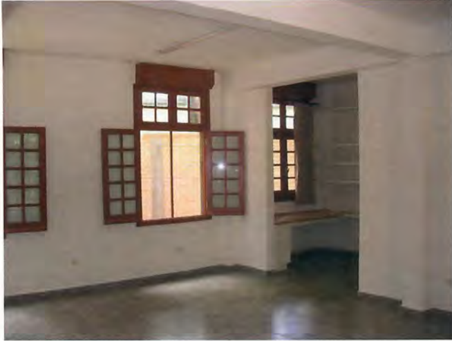
Figure 1.7 In-swing casement windows are commonly used in Madagascar
