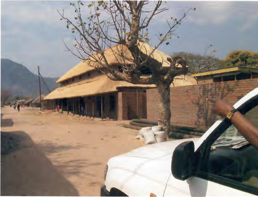
Figure 1.4 Contemporary use of thatched roofing in Malawi
