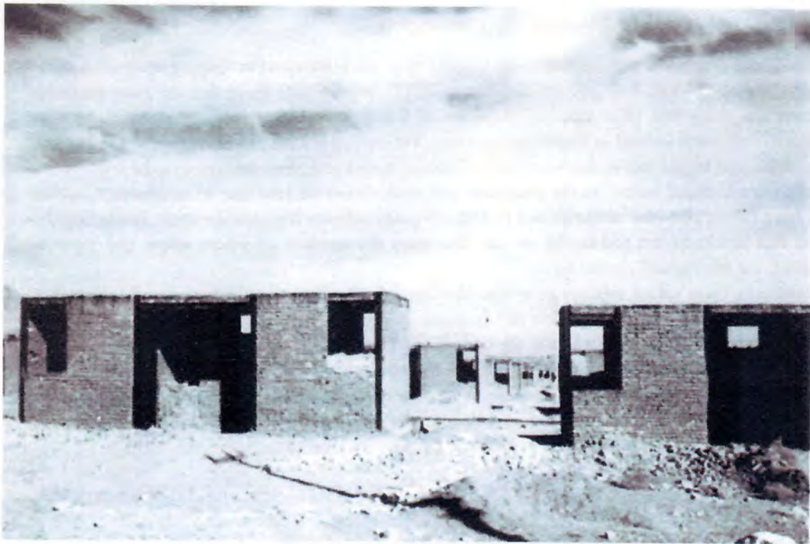
Figure 31.1 Housing project abandoned by the target population. Bojnurd earthquake housing reconstruction.
