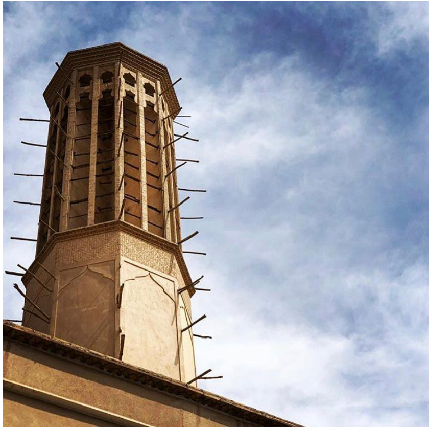
The wind capture tower of Bagh-e Dowlatabad house, Iran
