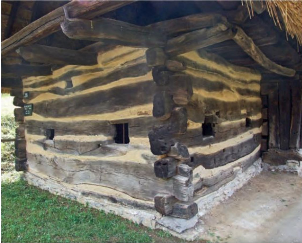
Log wall with clay, Austria
