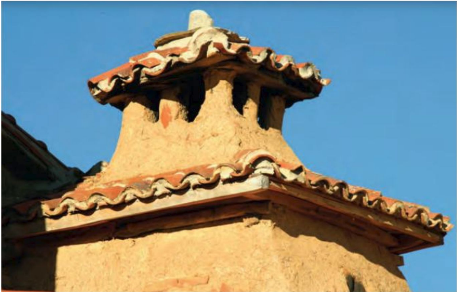
Earthen chimney, Spain
