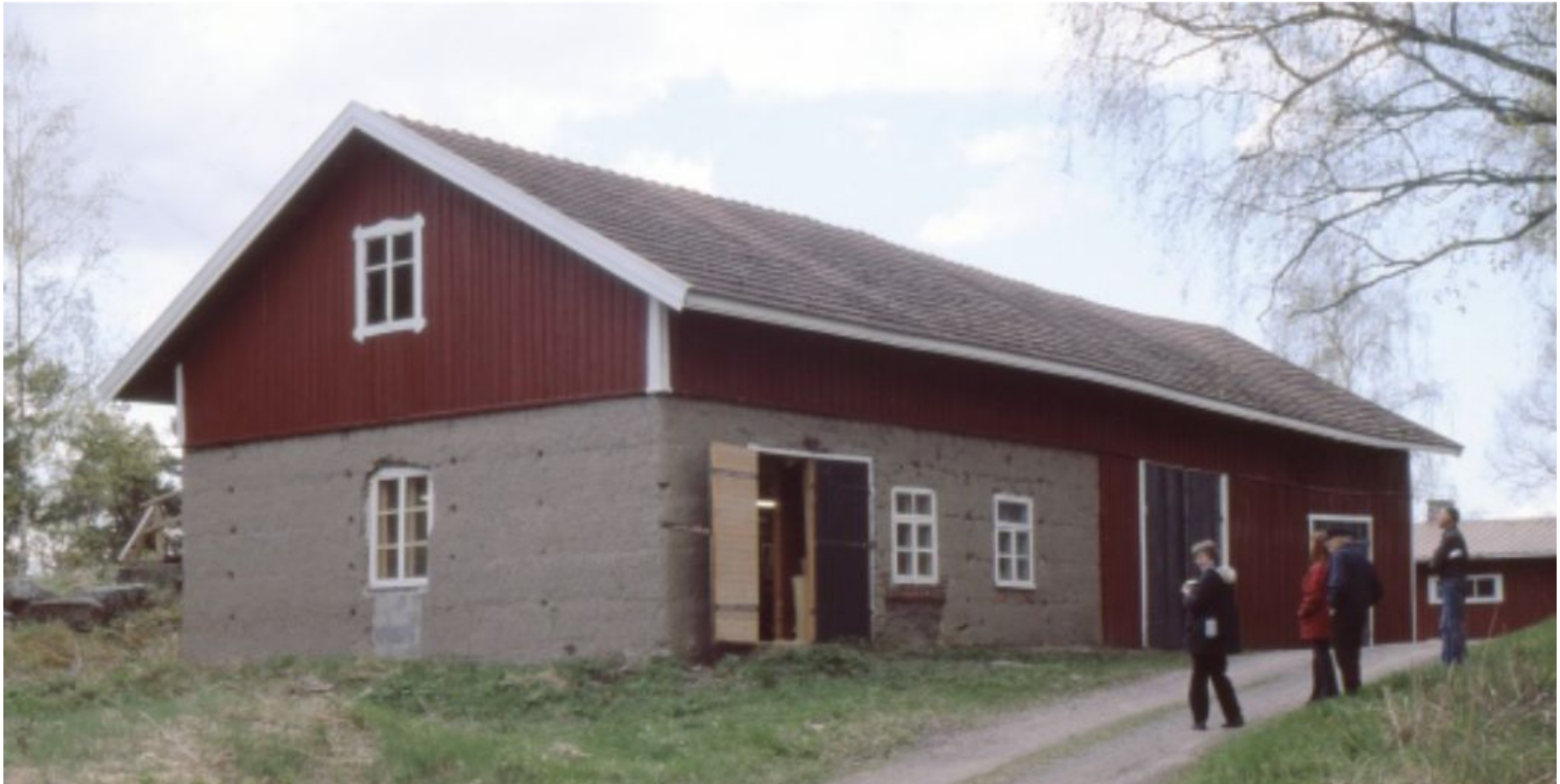
Barn with wooden and earthen walls, Finland
