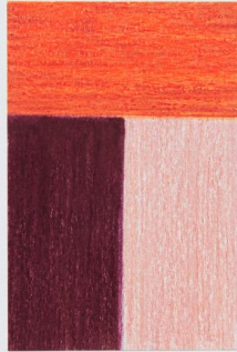
Cracked paint, Torii Gate
