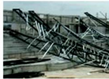
Figure 3.26: Illustration of possible consequence of too large rotations or displacements after stability loss.
