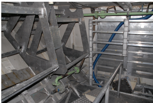
Figure 9: Empty store in the forward compartment
