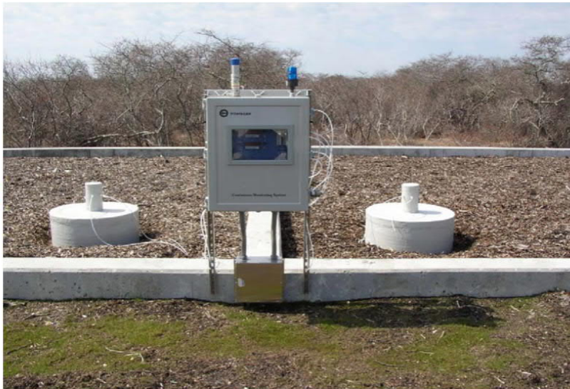
– Siasconset WWTF Biofilter for Odor Control
