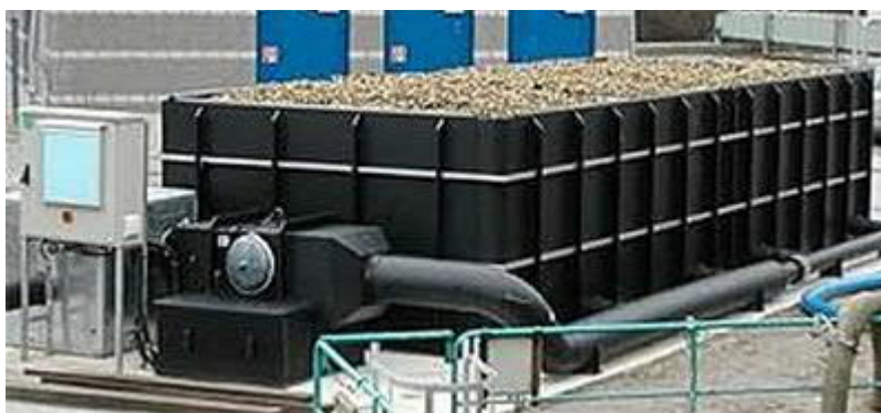
– Siasconset WWTF Biofilter for Odor Control
