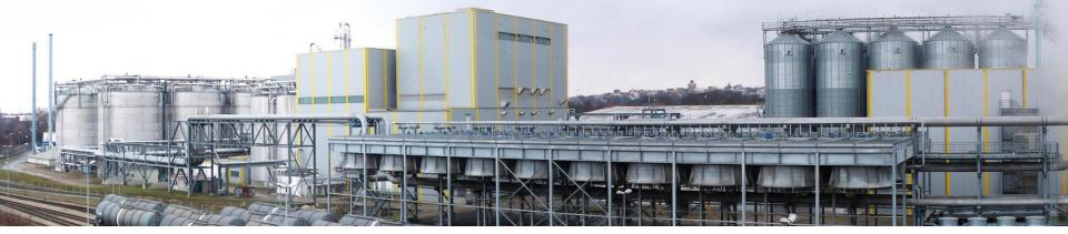
Bioreactors for ethanol production can be over 1000 m<sup>3</sup> (10<sup>6</sup> litres) large
