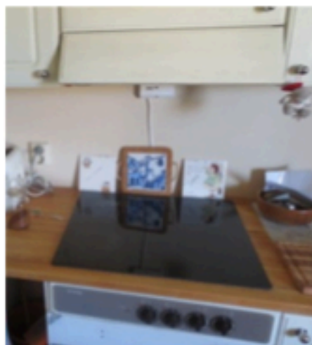
"Stove guard" that turns off the stove after a certain time and if there is nothing on it.
