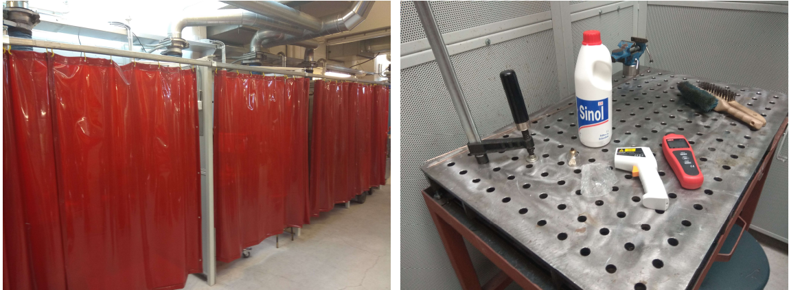
Figure 22 Testing stations at K2 shop, welding room.
