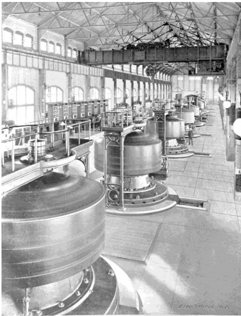
FIG. 11.—A VIEW OF THE TESLA ROOM, LOOKING SOUTH FROM THE VISITORS' GALLERY.
