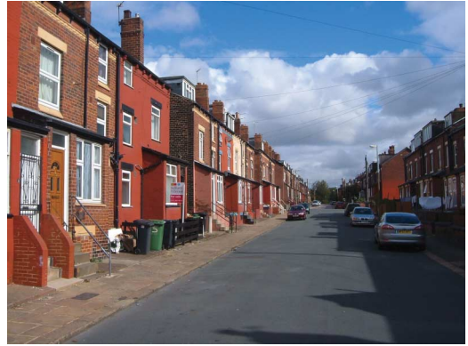
Figure 3 Copperfields Grove, Cross Green: the story of a street. Source: authors.
