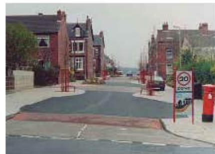
Figure 3.2 Gateway at western end of Methley Drive
