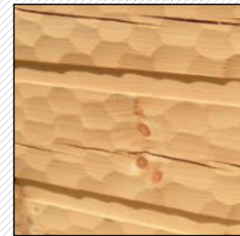
pine logwall with adzed finish
