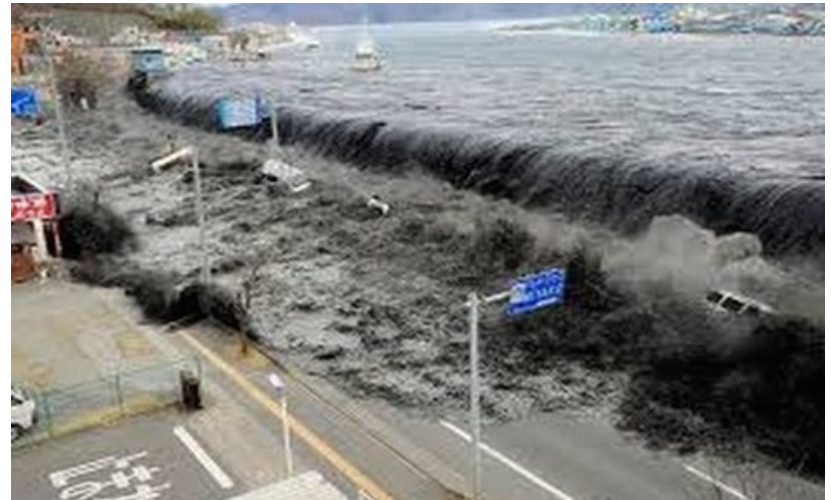
Although the impact of tsunamis is limited to coastal areas their destructive power can be enormous
