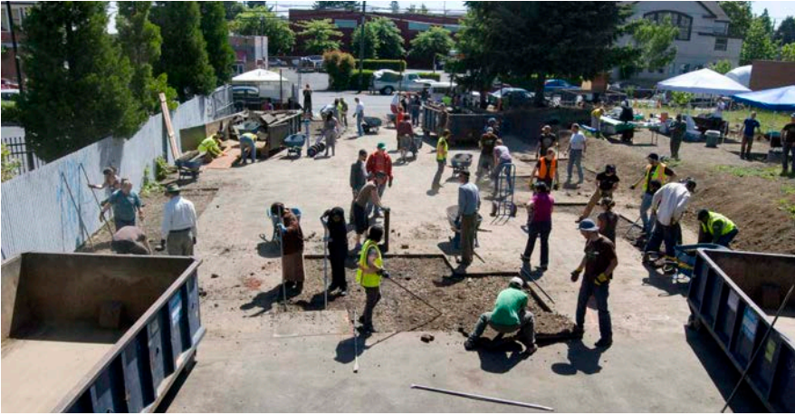
In Portland, US, nonprofit organisation Depave promotes the removal of unnecessary concrete pavement.
