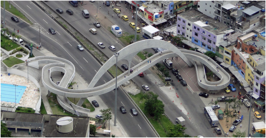
A footbridge designed by O. Niemeyer connects Rocinha, the largest favela in Rio de Janeiro, to a new sport facility.
