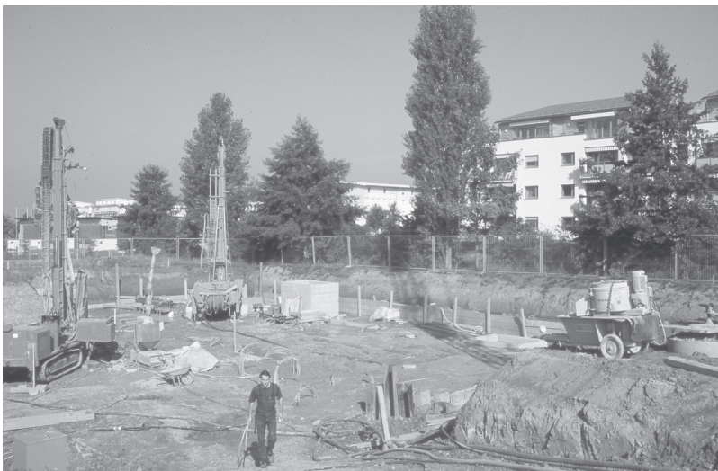
Figure 6.15 Construction phase of the first extension to 168 boreholes.
