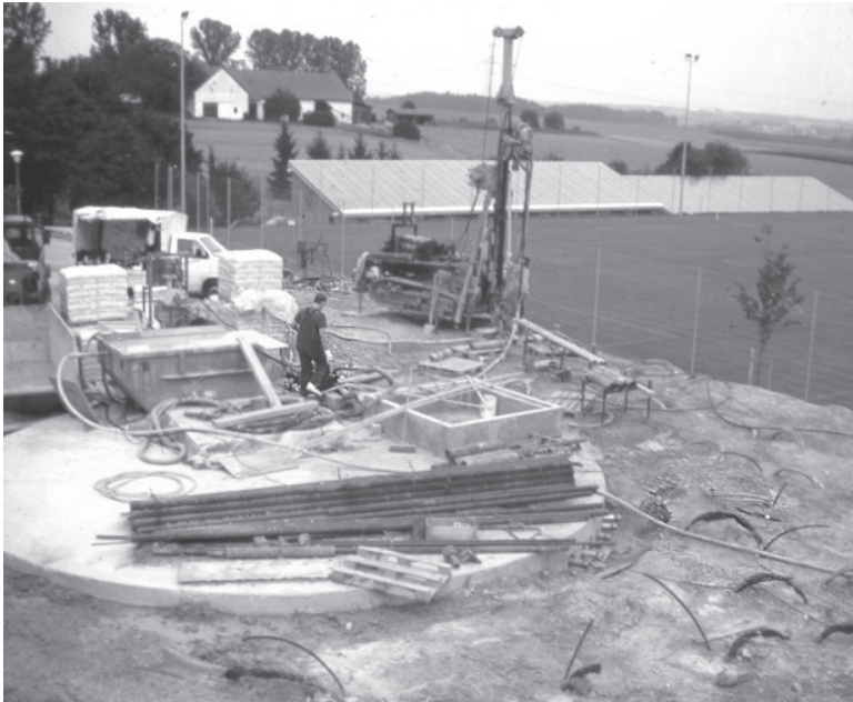
Figure 6.21 BTES construction surrounding the concrete tank.
