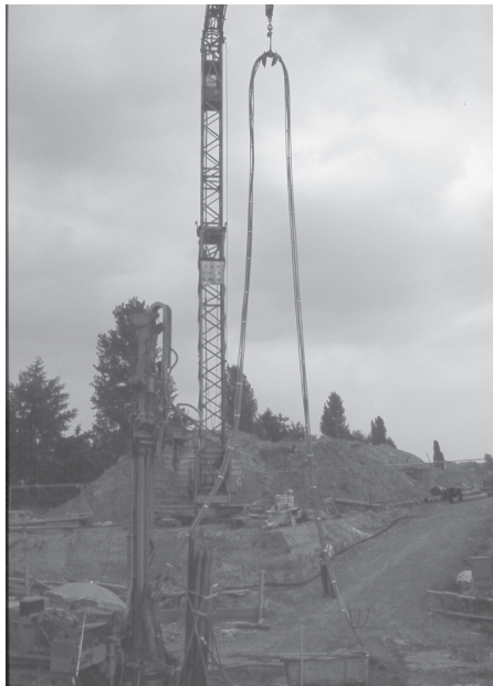
Figure 6.11 Installation of double-U-BHE at the BTES in Neckarsulm, Germany.
