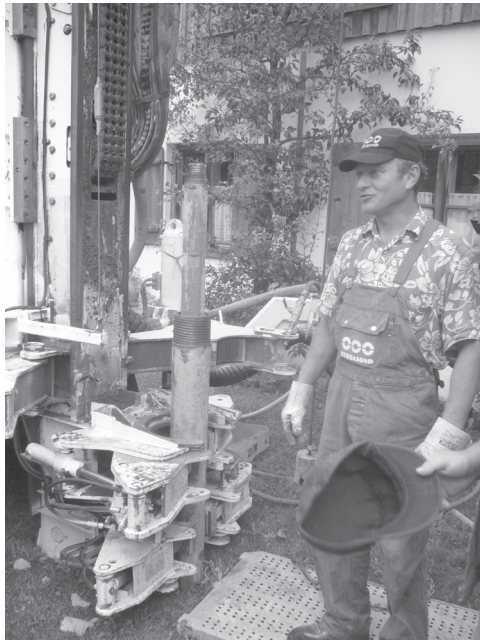
Figure 6.9 Drilling with casing.
