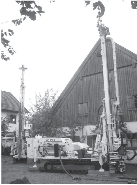
Figure 6.8 Double head drilling rig.
