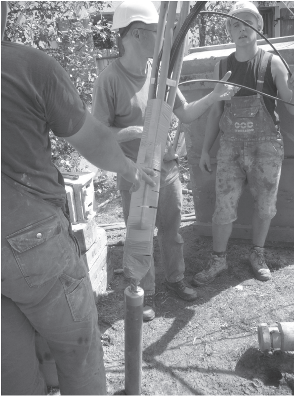
Figure 6.12 PE-X double-U-BHE with bottom weight.
