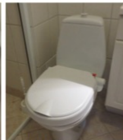
Heightened toilet seat.
