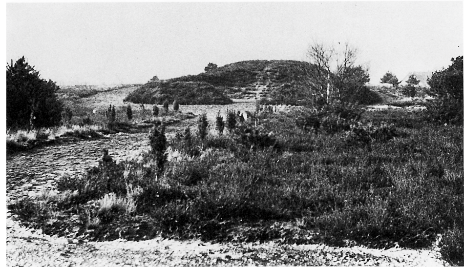
5. Mortuary in the Seelenfeld cemetery, shortly after its erection, ca. 1930
