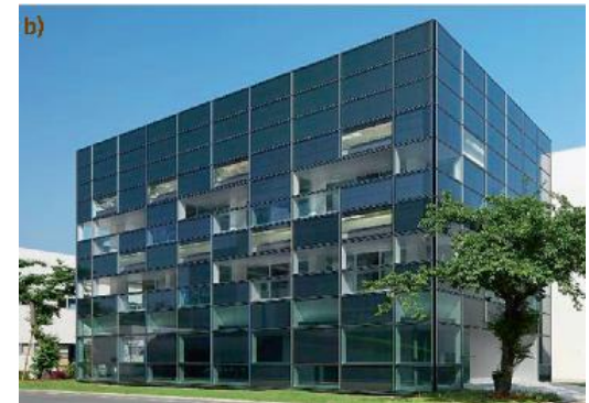
Building using OPV modules on the exterior walls and windows (Taisei Corporation)
