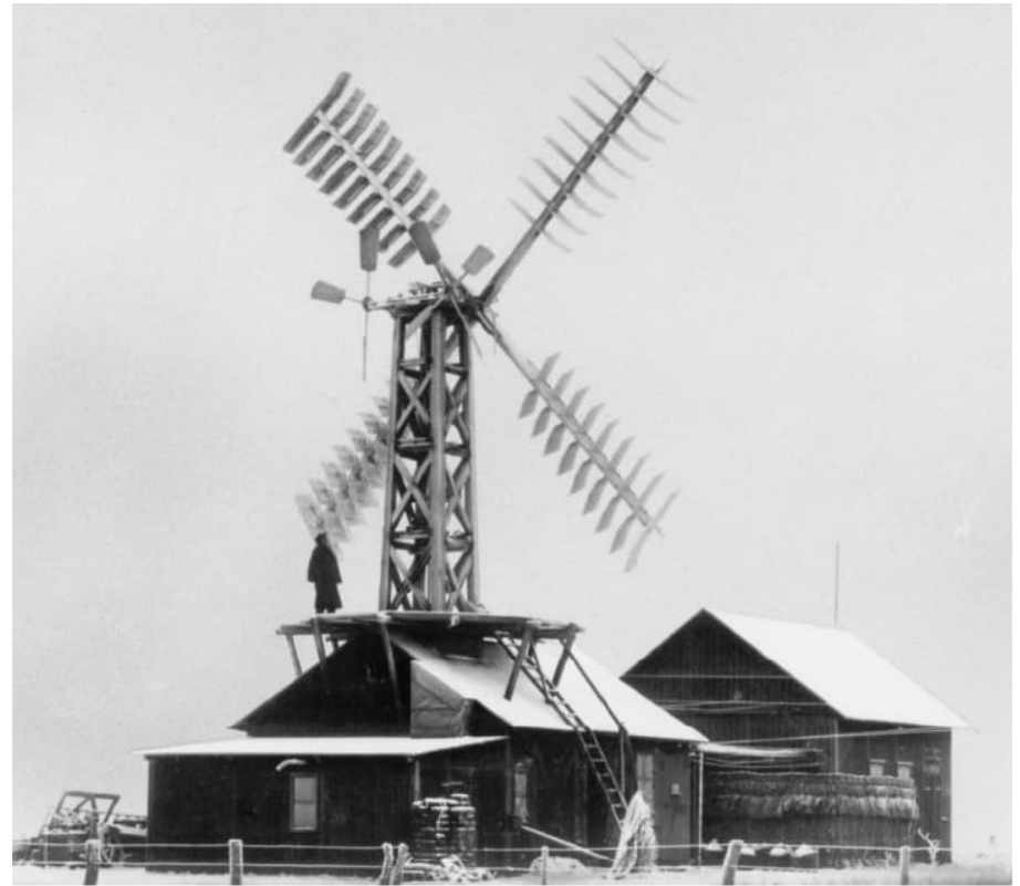
Fig. 2.1. Poul La Cour's first electricity producing wind turbine in 1891 in Askov, Denmark [1]
